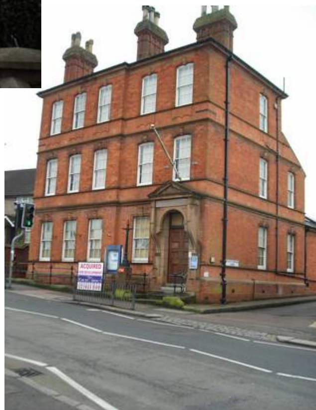
The former police station at Clay-Hill, Bushey, built in 1897 but I think possibly on the same site as the earlier one.
